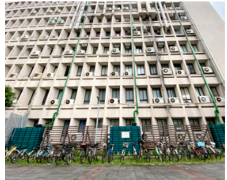
The rainwater storage system of the Second Engineering Building
