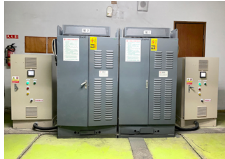
Elevator power recovery system
